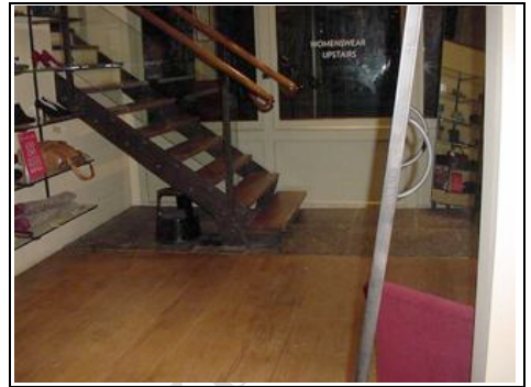
Customer's stairs to first floor
