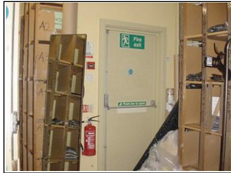
Fire exit to spiral staircase
