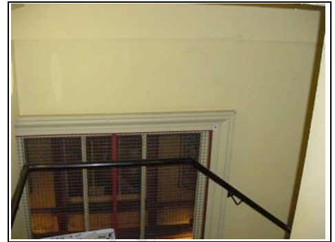
Window within staff staircase area
