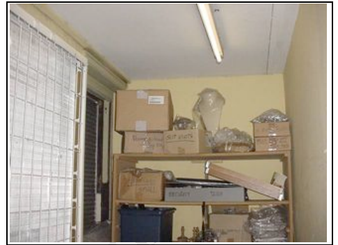
Ceiling in plant room
