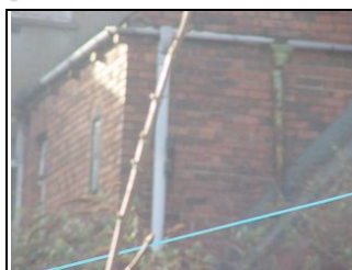
Gutters and downpipes
