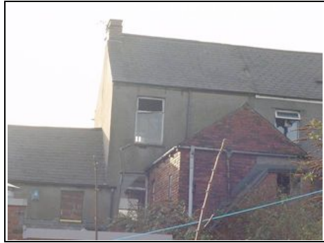
View of rear
