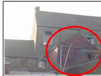
Rear two storey brickwork extension
