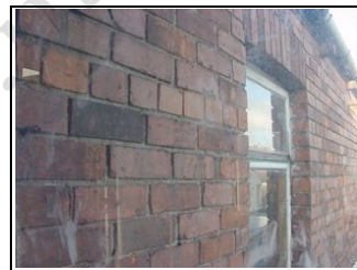
Brickwork rear extension
