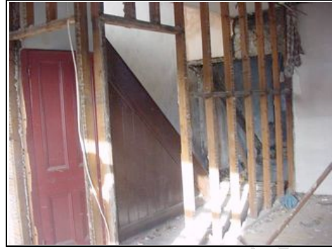
Studwork around staircase
