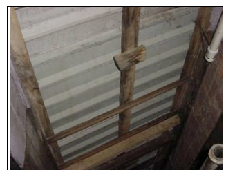
Underside of roof
