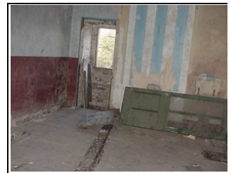
Looking at chimney and doorway
