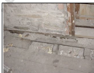
Floorboards missing
