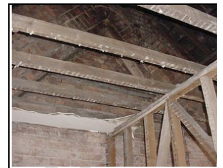
Unaffected roof timbers
