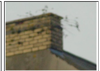
View of chimney
