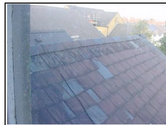
Top of slate roof
