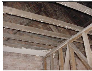
Looking at ceiling joists and roof
