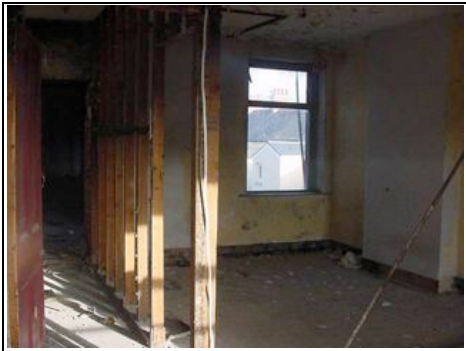
First floor room
