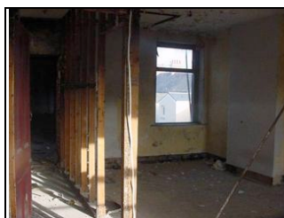
Studwork in place
