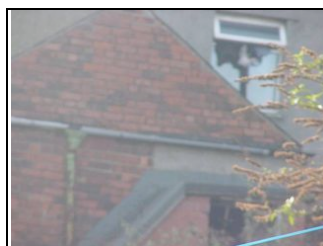
Roof over stairs
