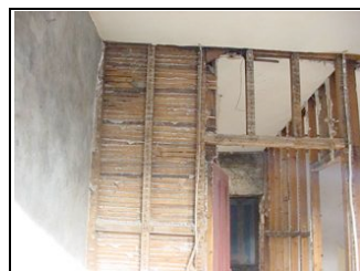
Some lath and plaster remaining.
