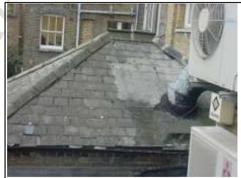
Felt repairs and lead tingles holding the slate on
