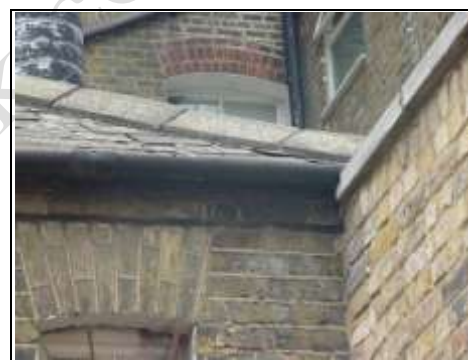
Fascias and soffits at low level
