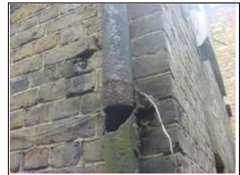
Broken downpipe
