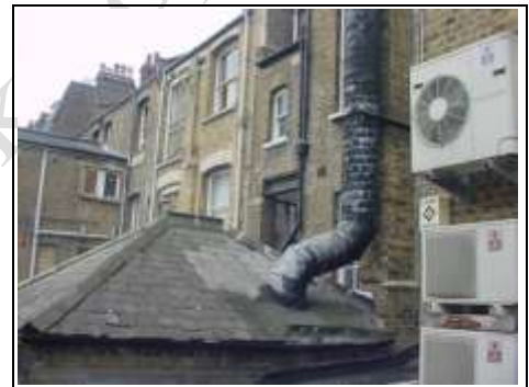
Extract flue not possible to clean hatches to these to allow
