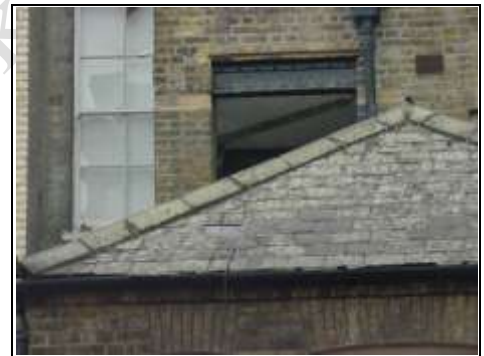
Low level rear roof
