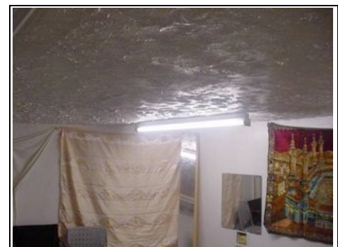
Textured basement/cellar ceiling finish
