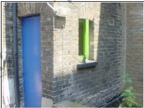
Rear terrace with access to toilet
