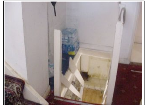
Access to basement/cellar
