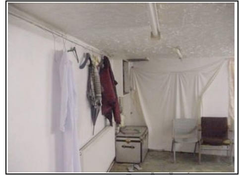
General view of basement
