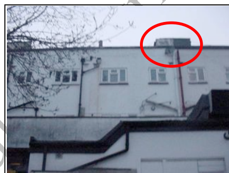
Rear of property high level area
