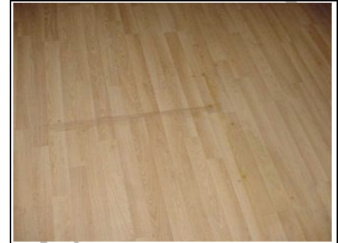
Marks to laminate shop floor
