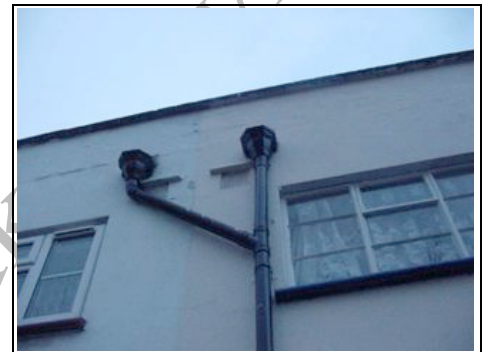
Hopperheads and downpipes
