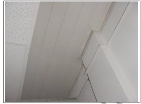
Cladding behind suspended ceiling in office
