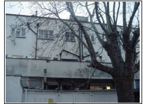
Tree to the rear of the property
