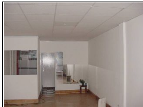
Rear of shop and right wall
