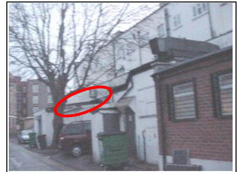
Rear conservatory roof
