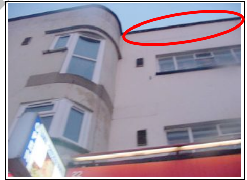
Hidden main roof
