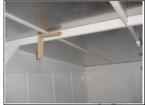
Polycarbonate roof internal view
