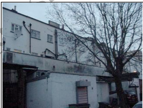
Render to walkway repainted
