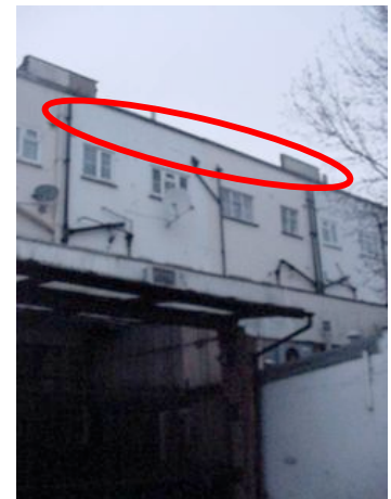
Rear main roof with parapet wall
