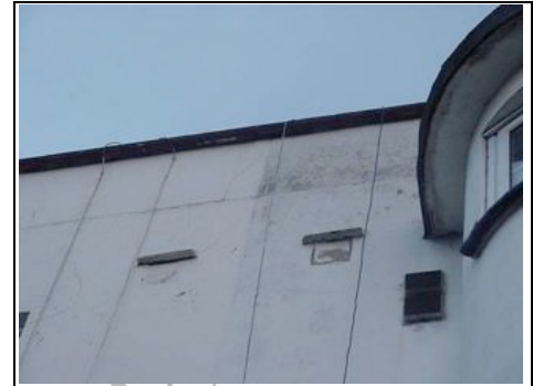
Hidden parapet wall
