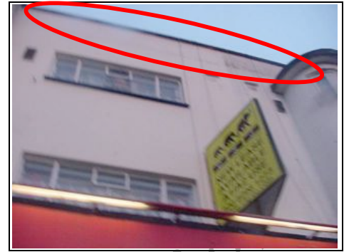
We have not viewed the roof
