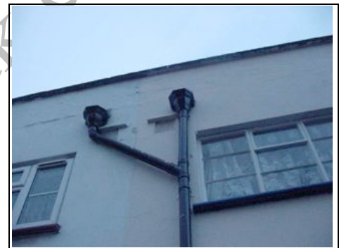
Box gutter and parapet wall to the rear of the property
