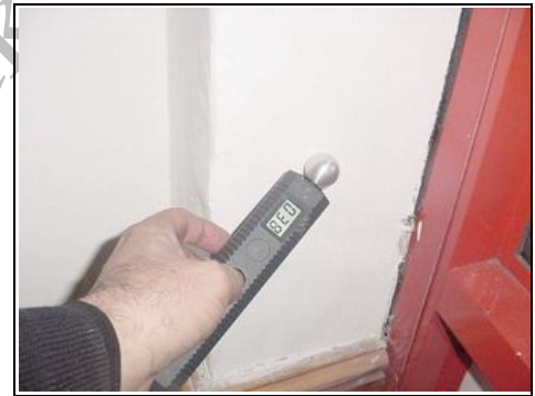
Testing for lateral dampness
