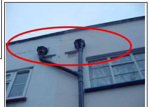
Hopperheads and parapet wall
