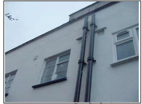
Soil and vent pipe to rear
